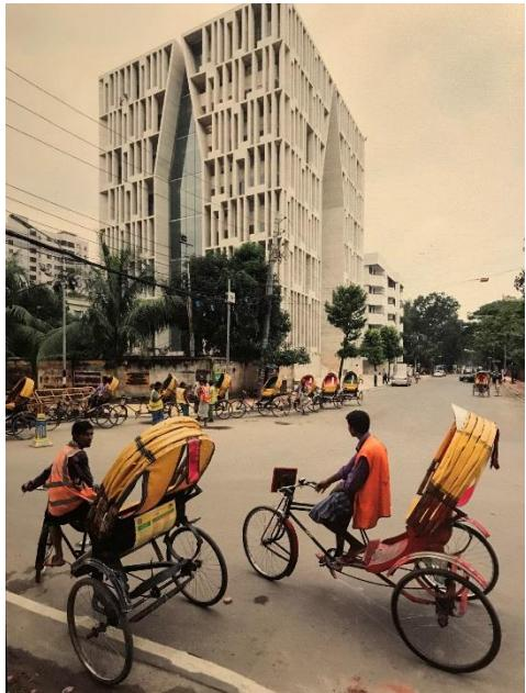
The Gulshan Society Mosque in Dhaka reimagines – and rearranges – mosque architecture with seven identical prayer halls stacked one on top of the other. The project's aim was to accommodate a large congregation on a small plot, while also providing an attractive landmark for the densely packed area. The building's outer pattern is an abstraction of a prayer in Kufic script.
